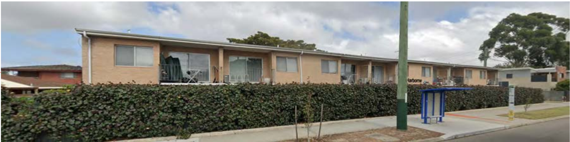
Apartments: 291 Harborne Street
