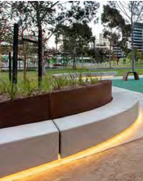
Concrete seating wall with timber top and integrated feature lighting
