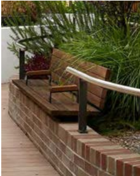
Brick seating wall with timber back and arm rest
