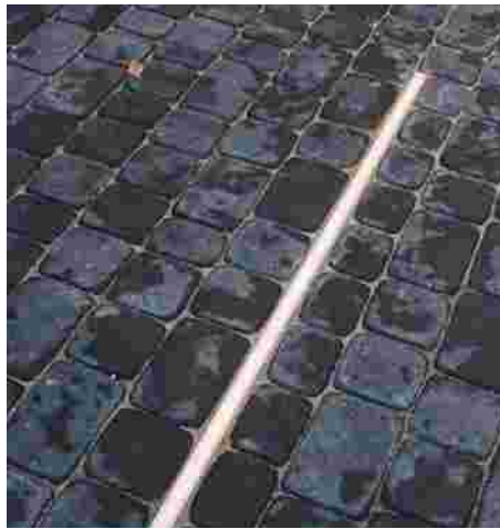
Description: In-ground Lighting
