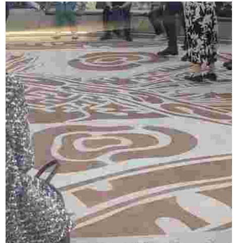
Description: Custom Concrete Pavement Product: In-situ Concrete Detail: Stenciled, stamped, sandblasted
