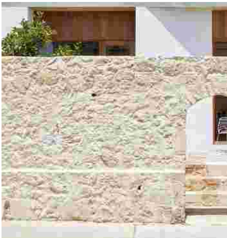
Description: Limestone Rubble Wall Colour: Natural Finish: Mortared
