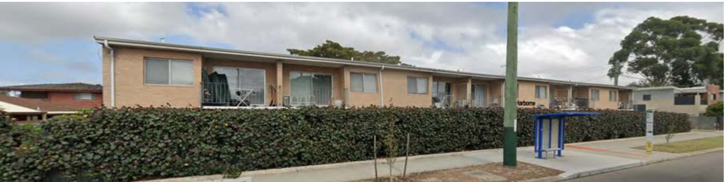
Apartments: 291 Harborne Street
