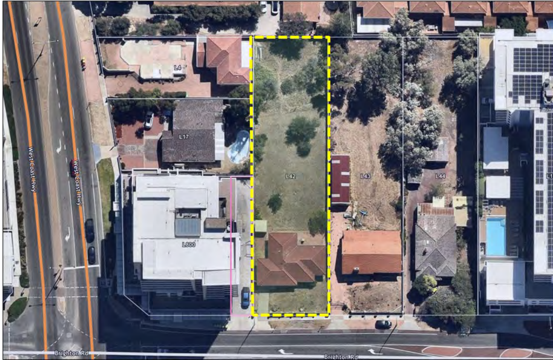
Site Aerial (MNG 2025)
