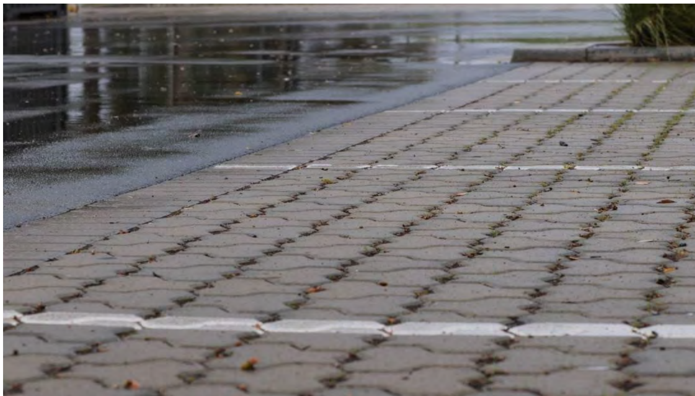
Figure 4.2 Vegetated areas and porous ground coverings are included in the development to aid in stormwater management.
