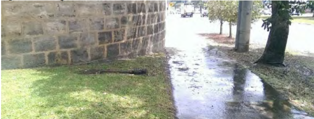
Figure 5 - Existing Water Connection
