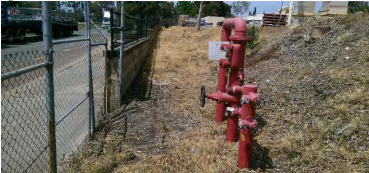
Figure 6 - Fire Booster
