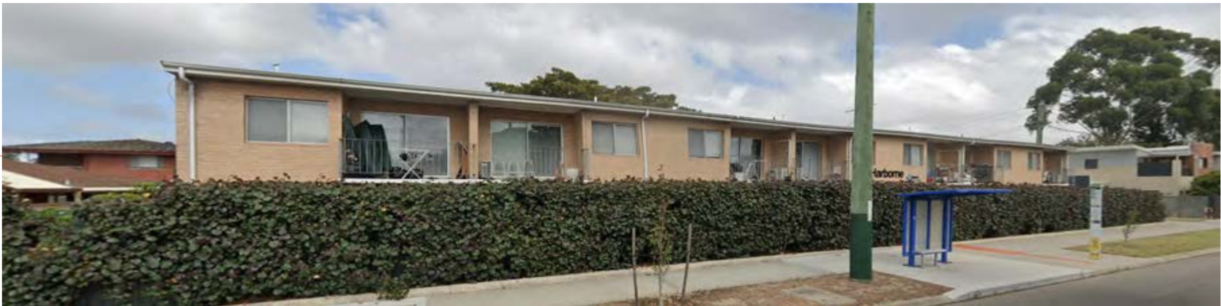
Apartments: 291 Harborne Street
