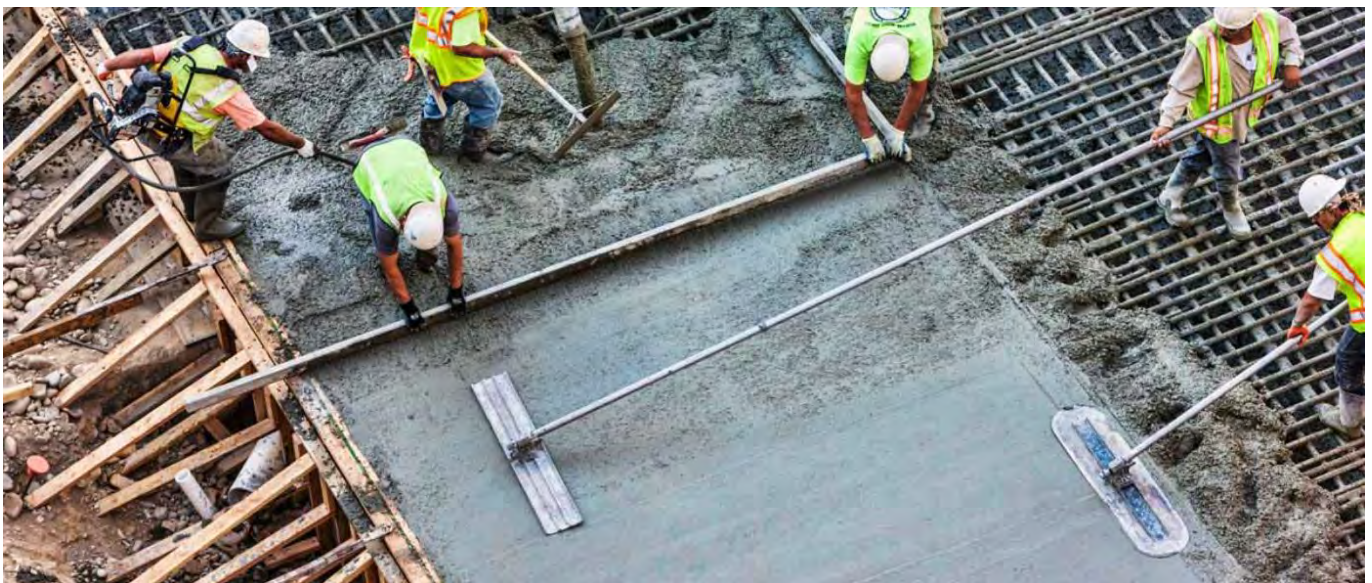
Figure 6.1 Construction site impacts will be managed during the project.
