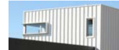
FEATURE CLADDING TO LEVEL 2,3,4 - Color bond trimdeck wall cladding in white
