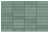
FEATURE TILING Green tile laid stacker bond
