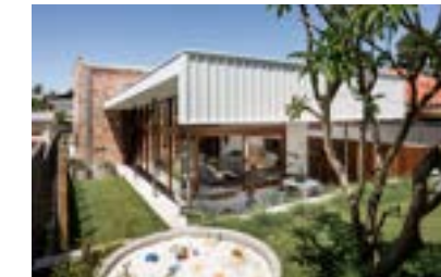
WINDOW FRAMES - Timber.Timber look window frames
