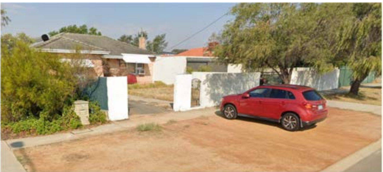
Figure 3 -The existing development on the subject land.
