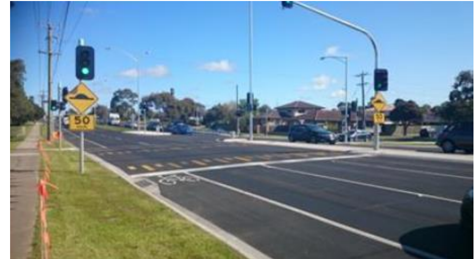
Figure 7b Street view of the raised safety platform in Belmont, Victoria.
