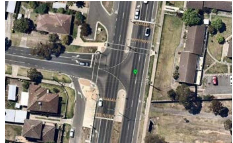
Figure 7a Aerial of the raised safety platform in Belmont, Victoria.
