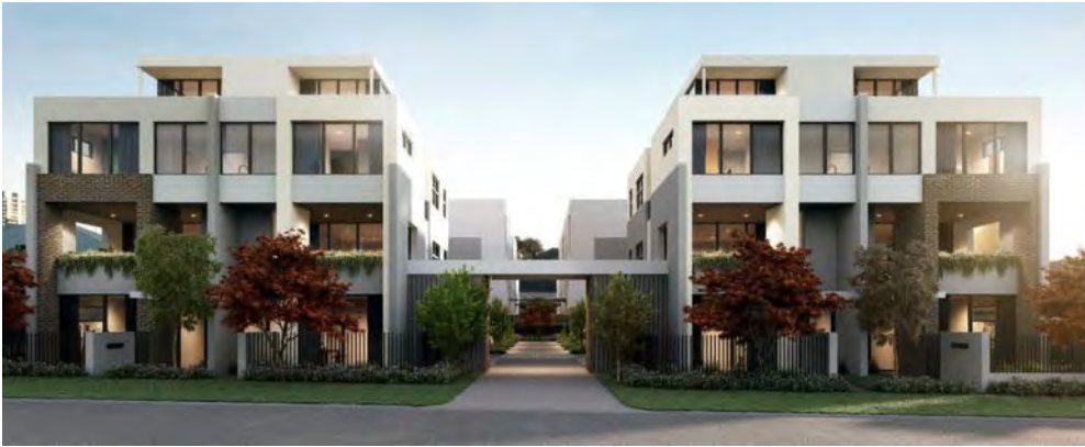
117-119 LOCKHART STREET 4 STOREY TOWNHOUSE IN CONSTRUCTION
