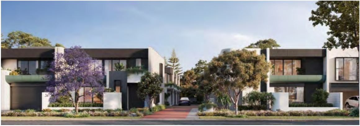
16 PHILP AVENUE 2 STOREY TOWNHOUSE IN CONSTRUCTION
