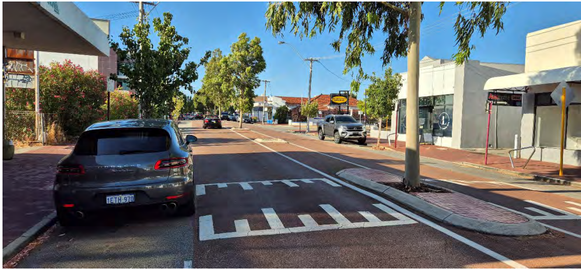
Figure 4: Northbound view along Oxford Street (adjacent to site)
