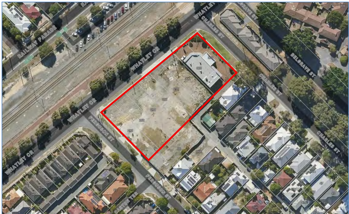
Figure 2: Aerial View (May 2025)
