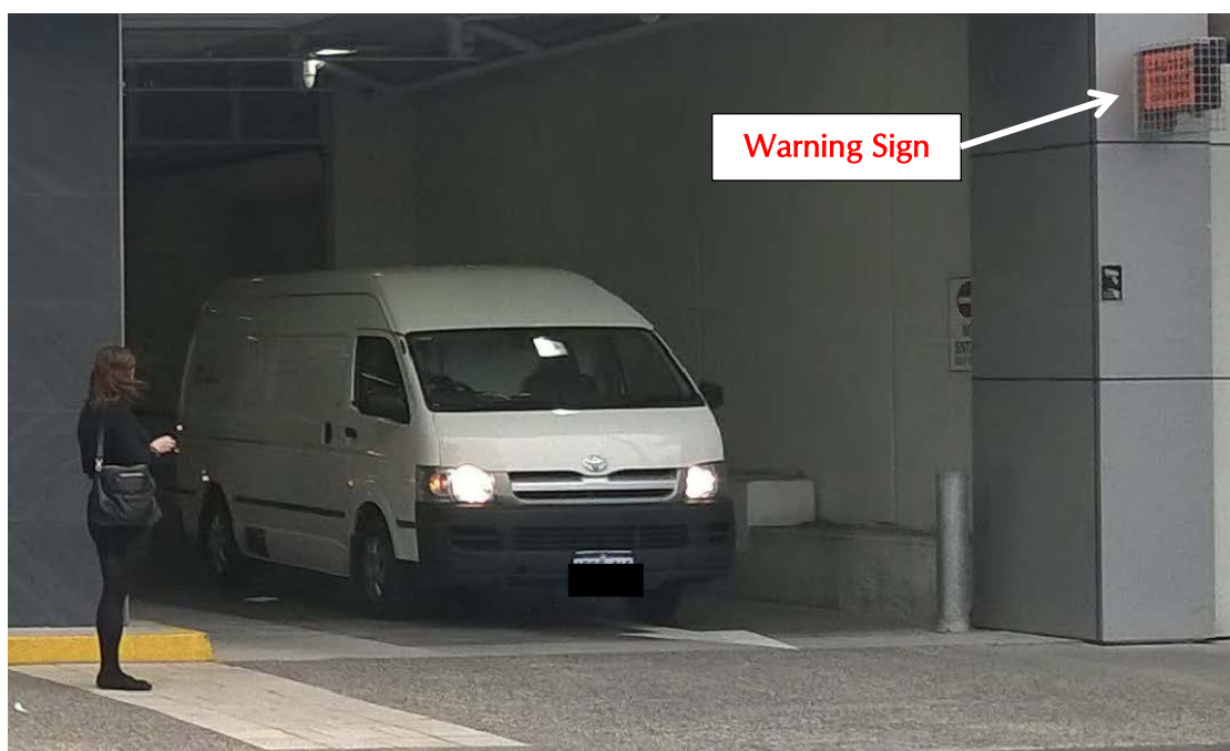
Figure 11: Example of illuminated pedestrian warning sign
