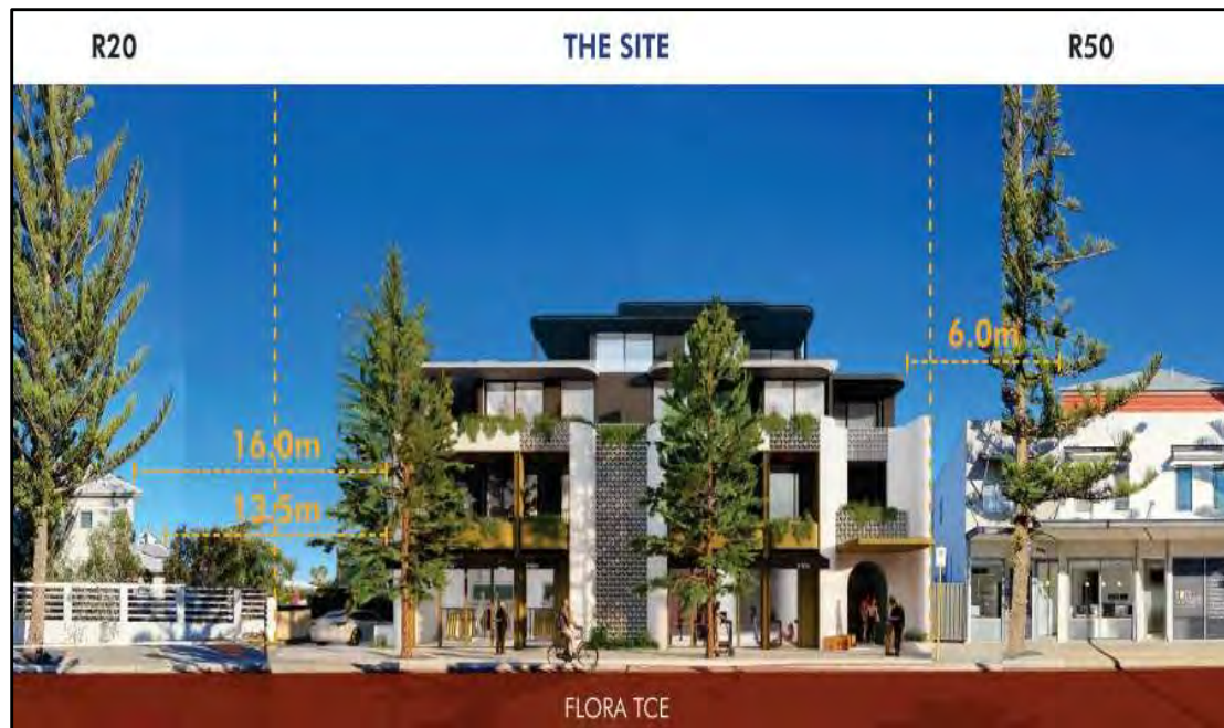
Figure 9 - The streetscape context of the development to the abutting southern and northern properties.
