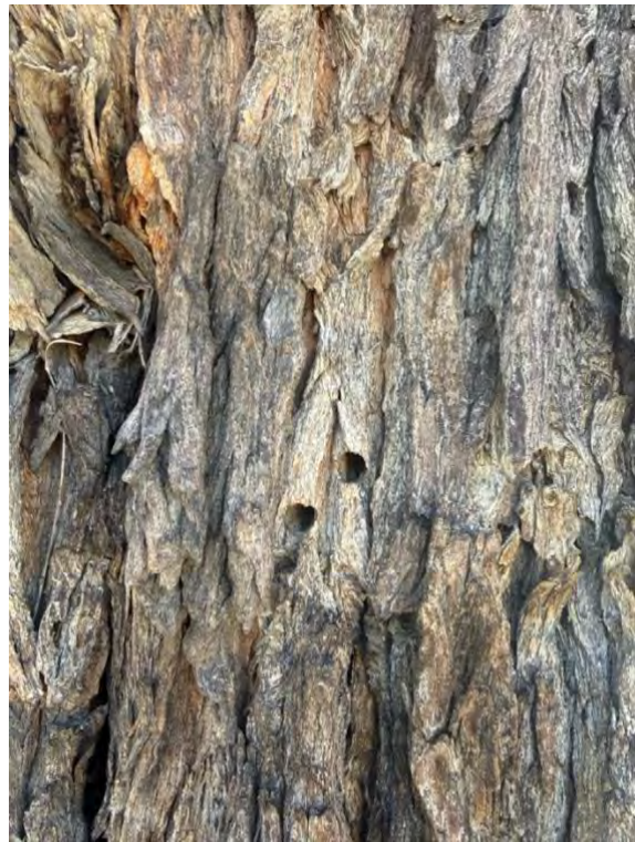
Figure 4 – Evidence of borer
