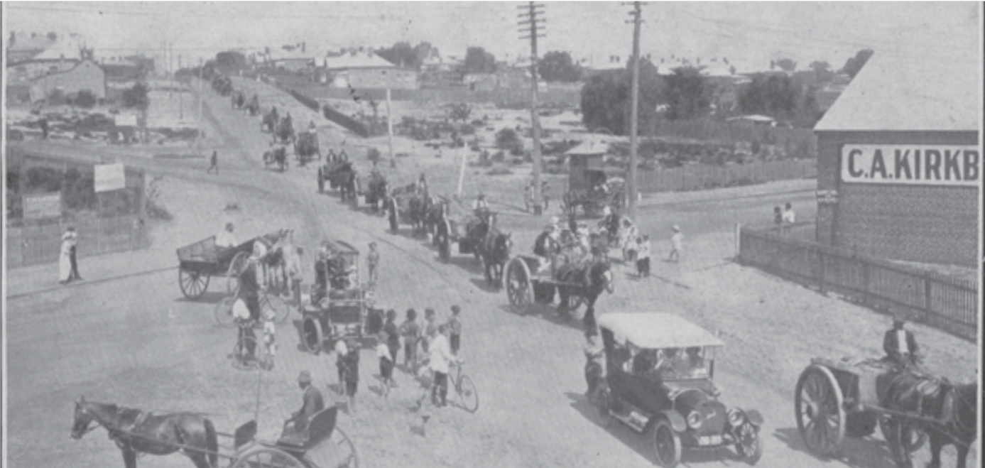
Carting the building material for ANZAC Cottage. 1916 (*)
