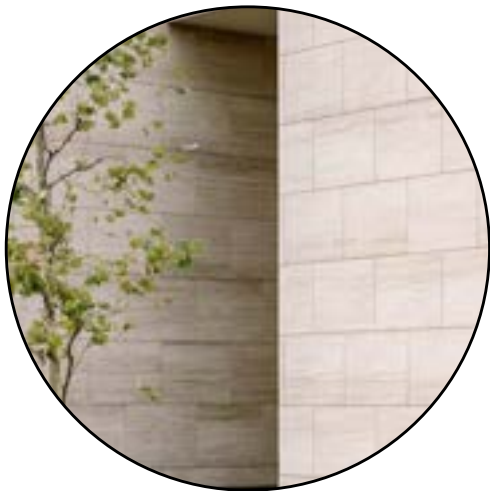
Limestone clad walls
