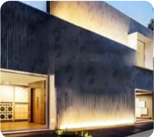
SOFFIT MOUNDED LINEAR WALL WASHER TO HIGHLIGHT ARTWALL
