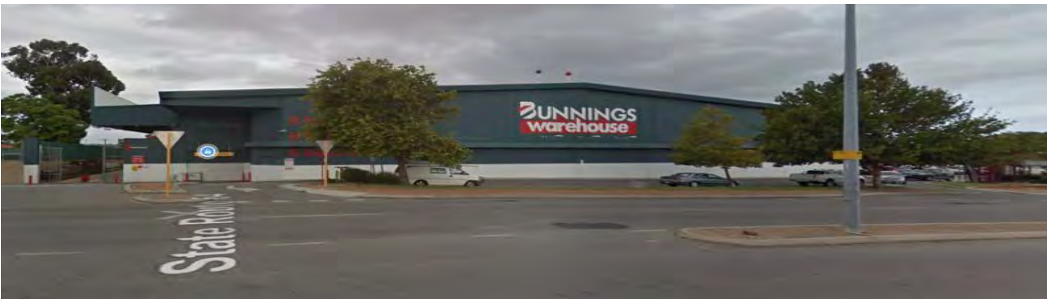
Commerical Development - Bunnings Warehouse - Corner Scarborough Beach Road & Odin Rd. Innaloo WA 6018
