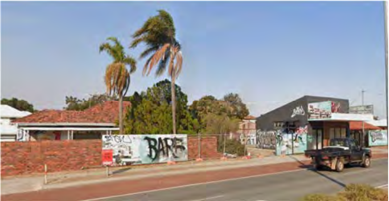
Figure 3 – The previous development on the subject land was run-down.
