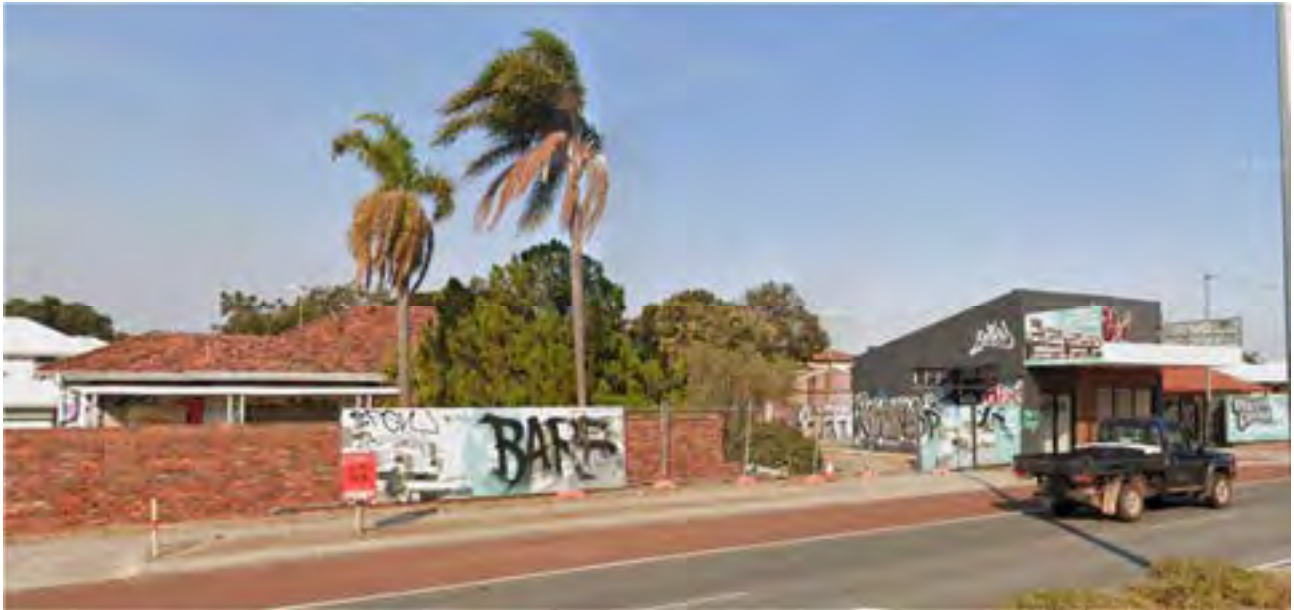
Figure 3 – The existing development on the subject land, which is run-down.
